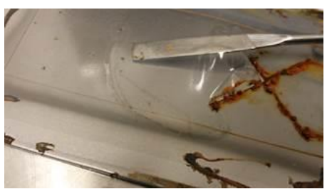
Figure 7: Loss of adhesion after 300hrs exposure to the B117 salt fog cabinet.
